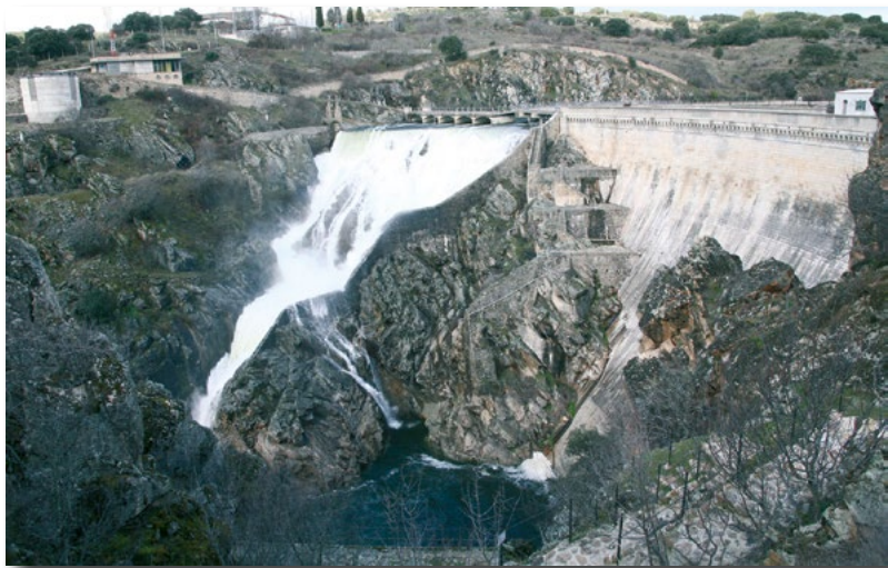
Spillway of the El Villar Dam.
