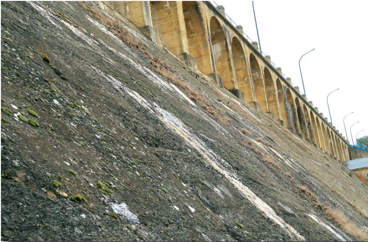
Study of the Villameca dam.
