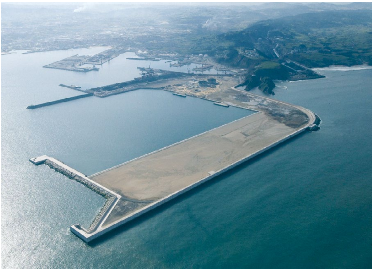
Figure 5. Project for railway access to the north quay (port of Gijón). Aerial view of the quay.
