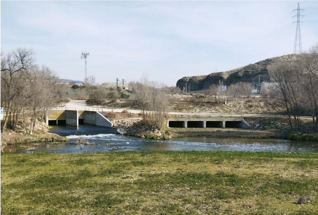
Spillways of the La Gavia WWTP and La Gavia stream, on the left bank of the Manzanares river.
