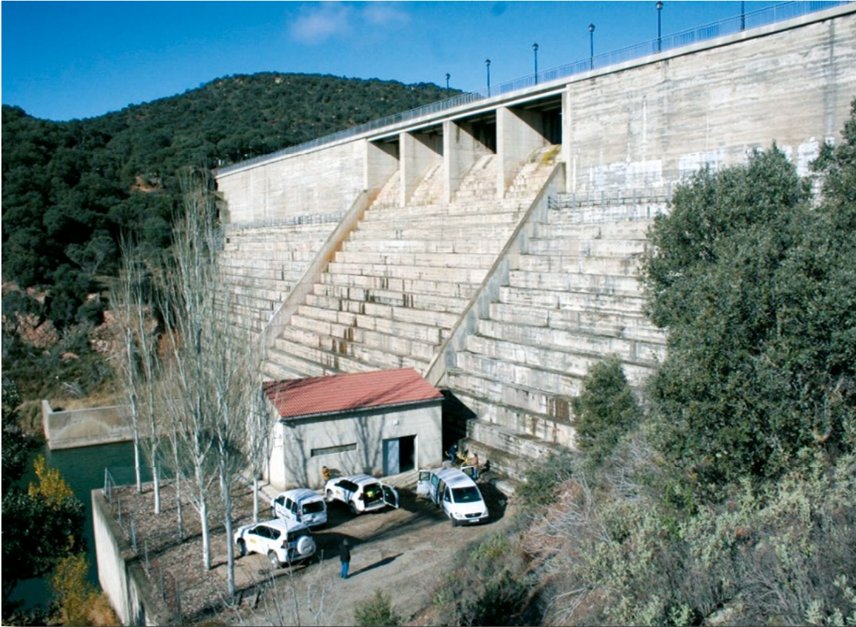
Figure 6. Characterisation of the foundation on the left abutment of the El Atance dam.
