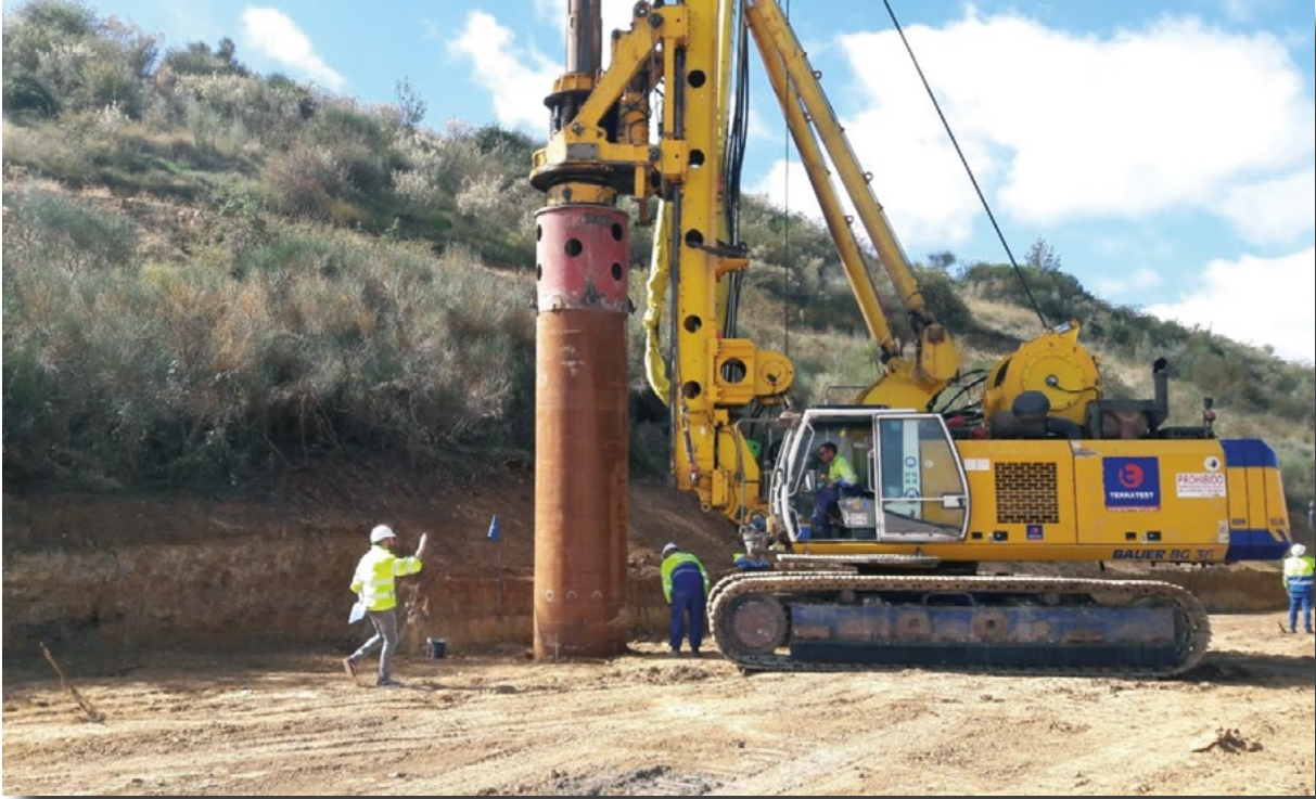
Execution of a pile screen for the correction of instability.
