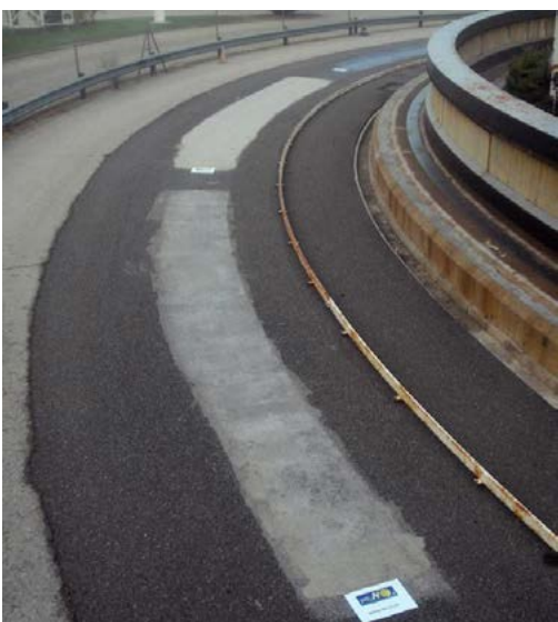
Implementation of photocatalytic products on a test track
