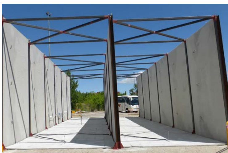
Construction of the double "street canyon" for pavements and façades
