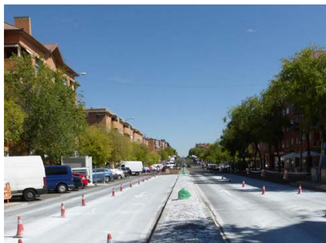
View of the road with the photocatalytic product applied
