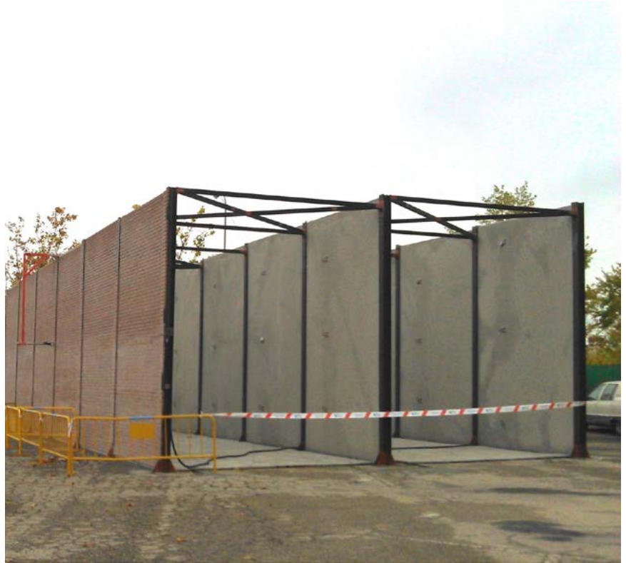
Street canyon brick wall used to measure \text{NO}_x and continuous weather parameters
