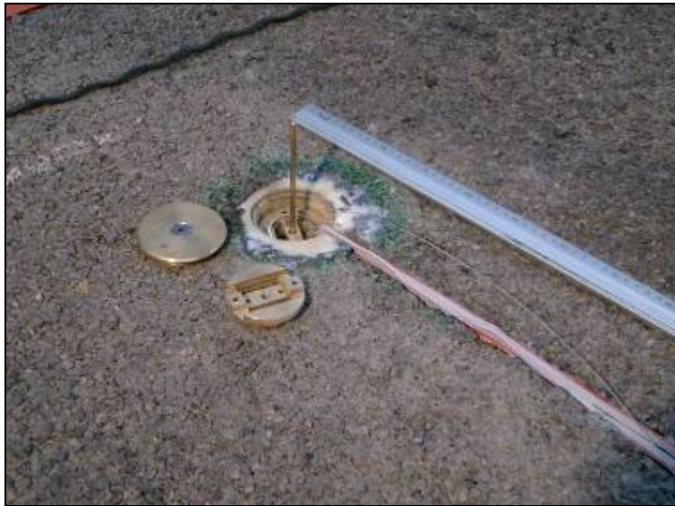
FIGURE 2 Installation of multi-depth deflectometers
