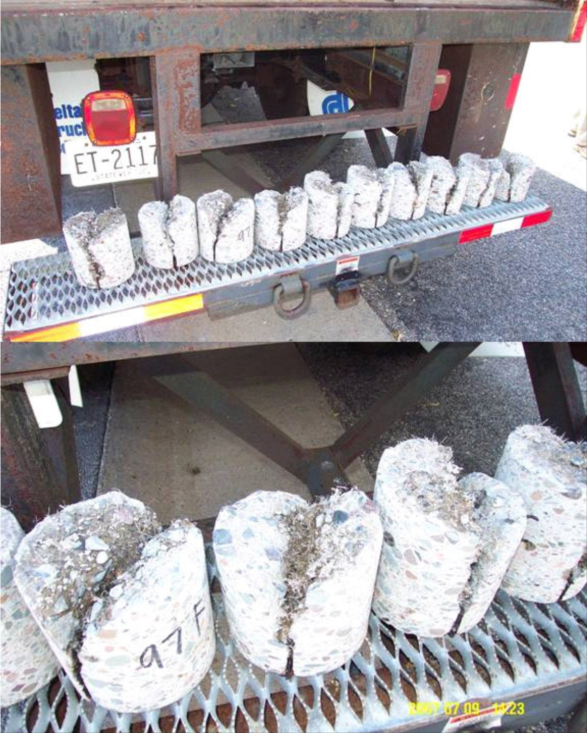
FIGURE 12 Condition of Concrete Cores at the Asphalt Interface.
