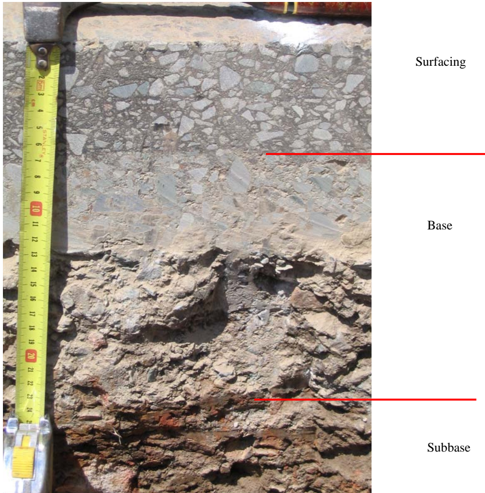
Figure 3: Photo showing the pavement surfacing and test pit.
