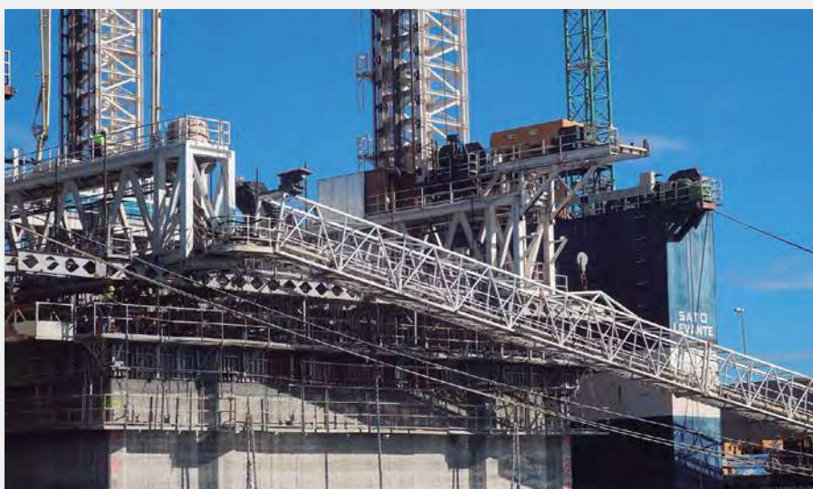
← Floating caisson fabrication.
