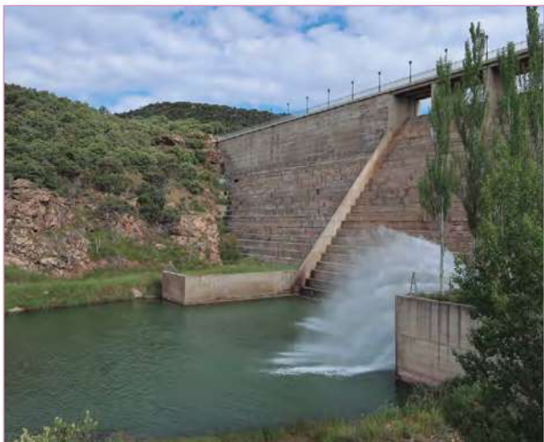
Analysis of the concrete for the Atance Dam.
