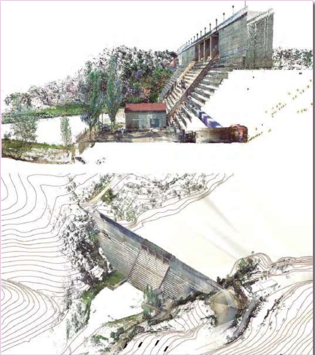
Point cloud of the 3D scan (above) and its geolocation in the BIM environment (below).
