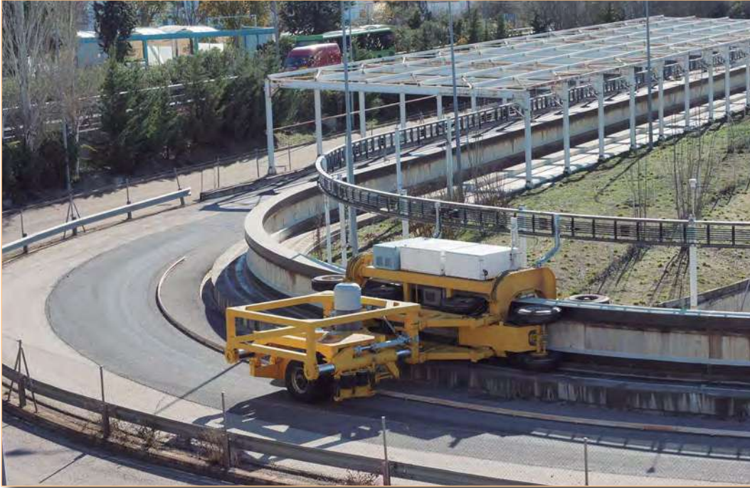
Accelerated pavement test track of CEDEX.
