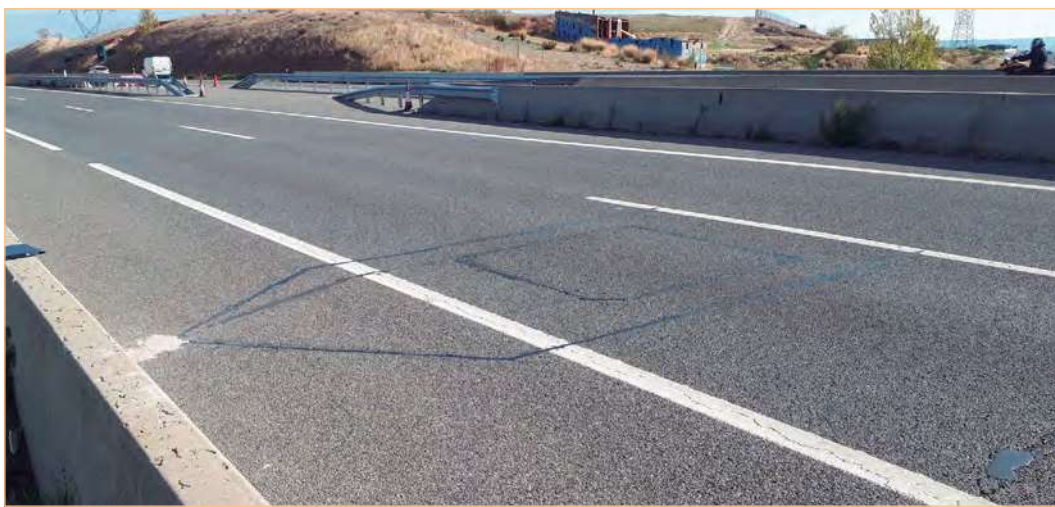
Piezoelectric-type weigh-in-motion system on the A-1 motorway in El Molar.
