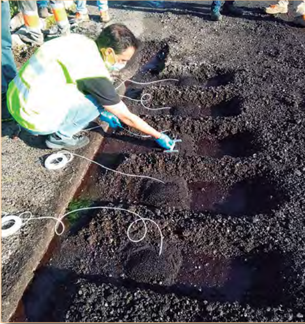
Placement of sensors in the pavement.
