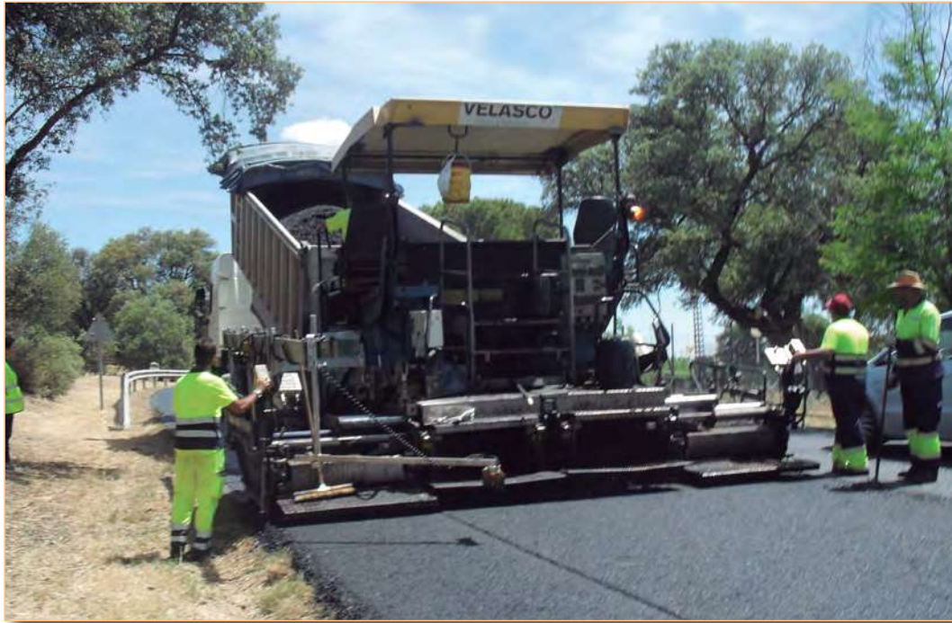
Laying of a low-temperature mixture.
