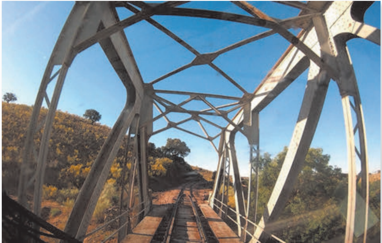
Line Almorchón-Alhondiguilla on which the GATE4RAIL project was executed.
