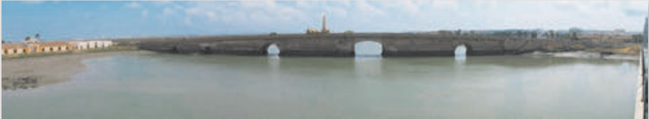
Inspection of the Zuazo bridge (Cádiz).
