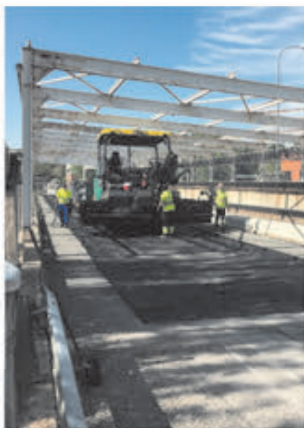
Placing bituminous mixture
