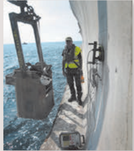
Corrosimeter: measurements in situ .
