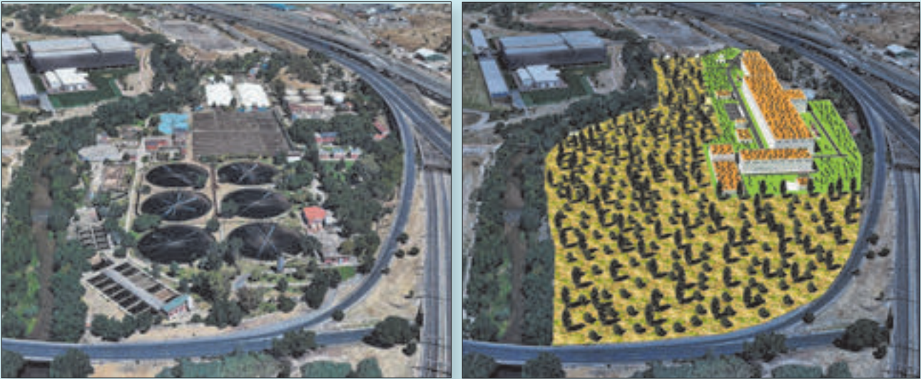
La China sewage treatment plant. Left: current plant. Right: Three-dimensional view of the proposed new plant.
