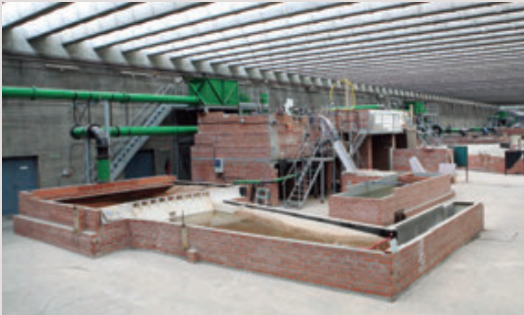
General view of Hall I (left) and Hall II (right).
