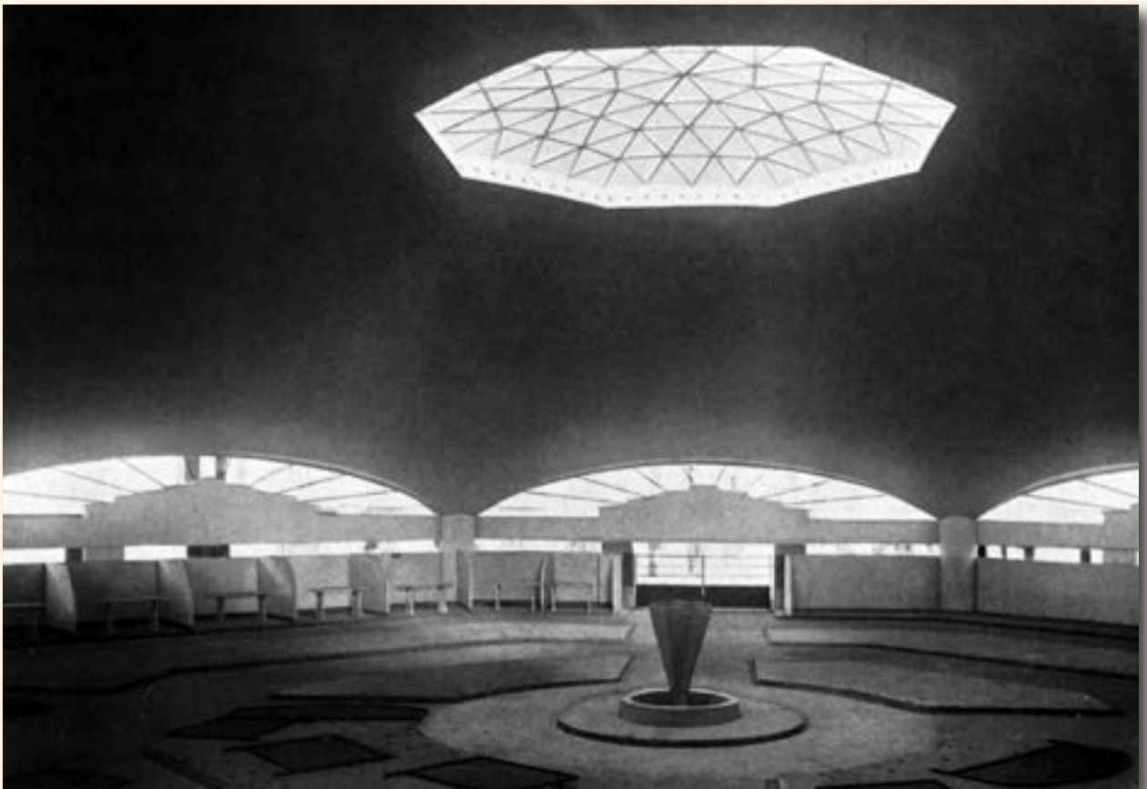
Images of the market of Algeciras, by Eduardo Torroja in the monograph E. Torroja. His Works. 1926-1936 . Madrid, CEHOPU, 2019.
