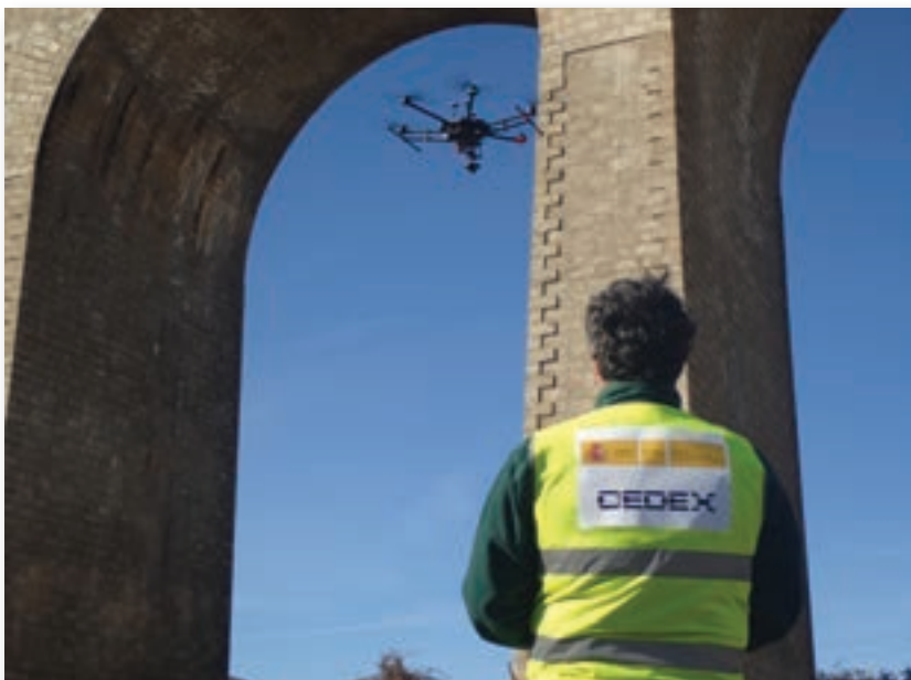
Structural inspection of a railway bridge.
