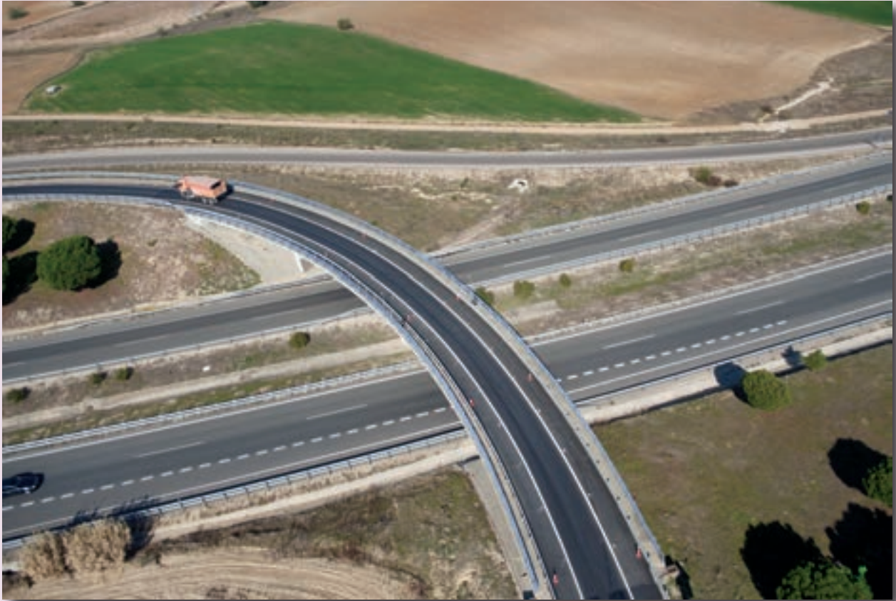
Dynamic tests have been carried out on an overpass structure.
