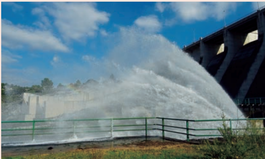
Howell discharge valve in Bellús reservoir.
