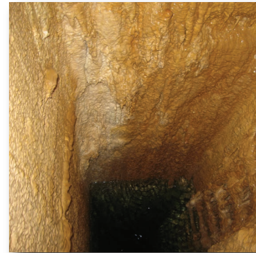
Carbonate crusts in a well.
