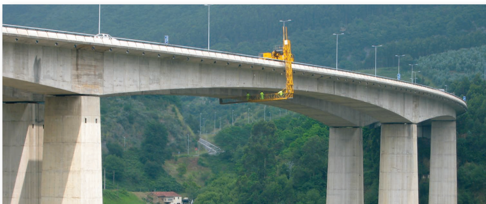
Inspection of the A8 bridge over Agüera estuary.
