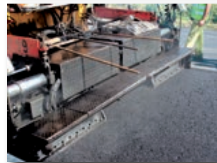
Laying and compaction of asphalt mixtures with NFVU crumb rubber.
