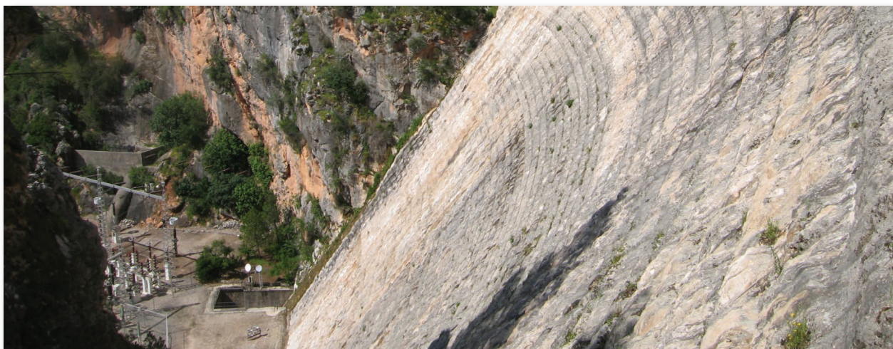
Downstream slope, Tranco de Beas dam.
