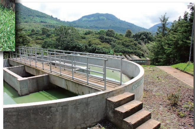
Wastewater treatment plant (El Salvador).
