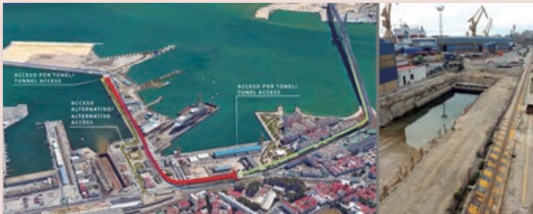
Figure 5. Access to the new terminal of the port of Cádiz.
