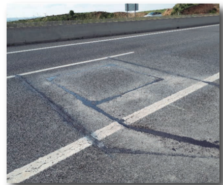
Final appearance of the weight sensors and the induction loop once installed on the roadway.
